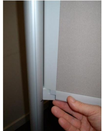
and then fix the top of the board by securing another peg downwards.
